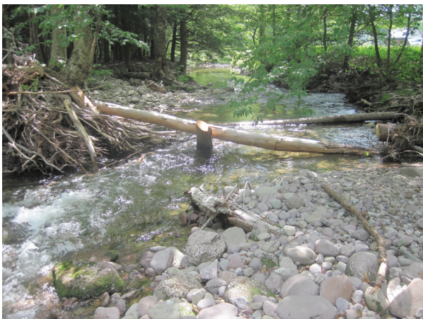
Large woody debris causing partial reroute of main channel (A60)
