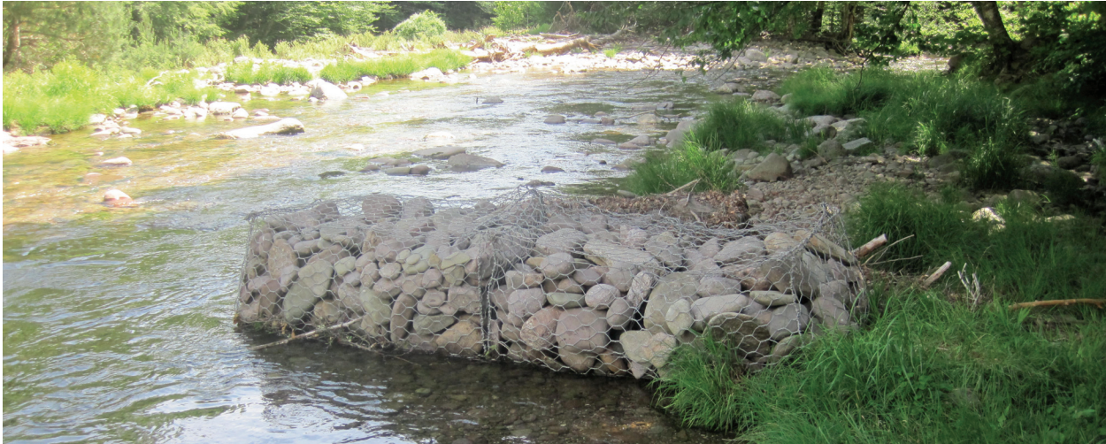
Gabion basket on right bank (A51)
