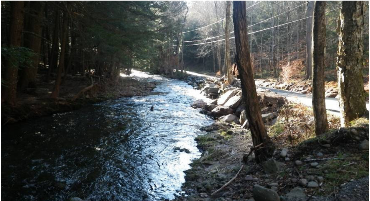
Recently constructed stacked rock revetment adjacent to Denning Road. (IMGP1523)
