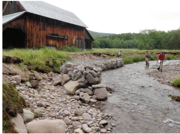
Gabion baskets placed on right bank to protect barn (B27)
