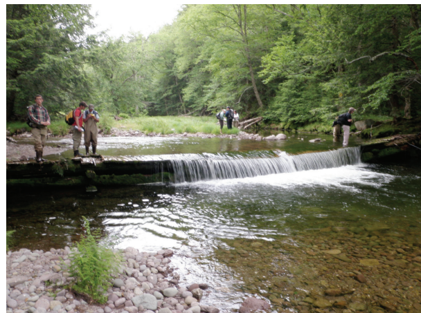
Looking upstream at wooden dam at station 46,110 (B34)
