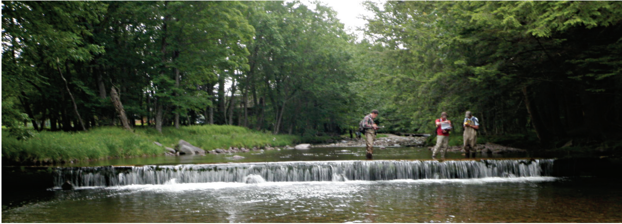
Looking upstream at wooden dam at station 45,760 (B46)
