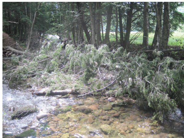
Obstruction causing erosion on right bank (A64)
