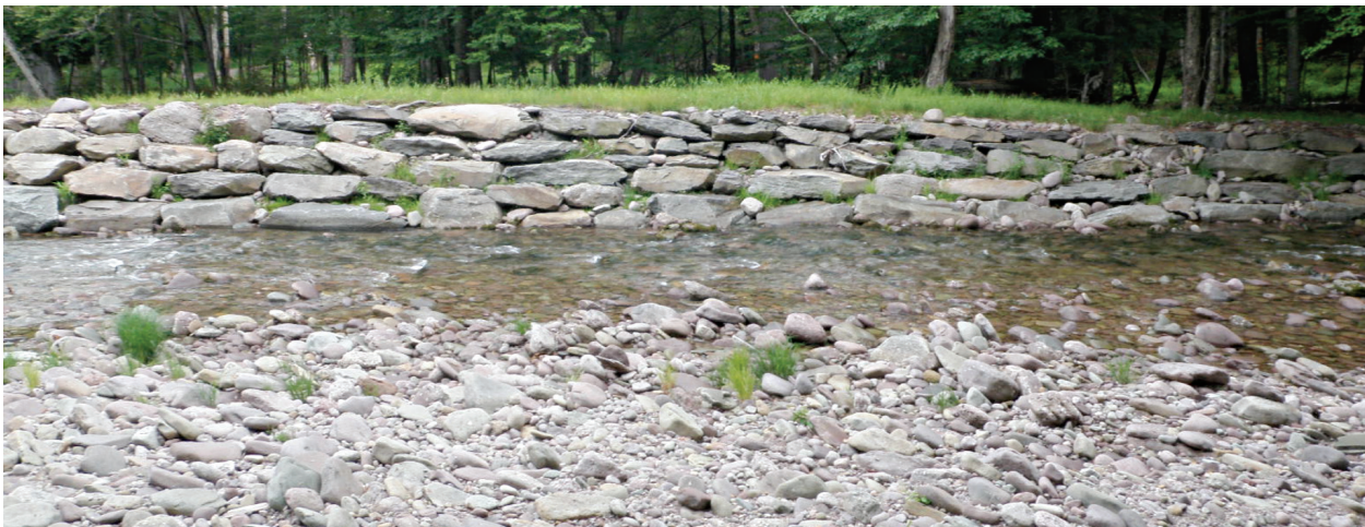
Stacked boulder revetment on right bank (B68)
