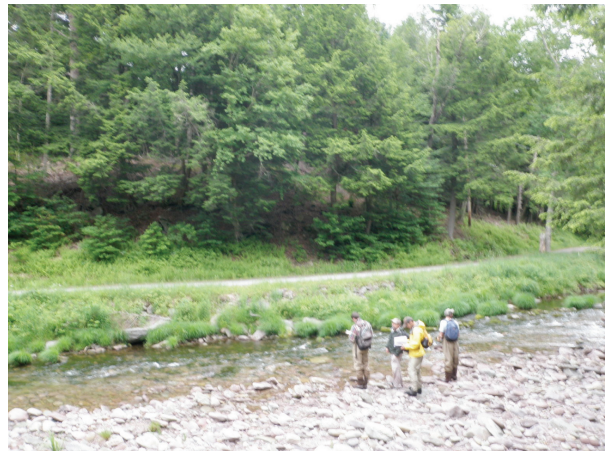
Cobble berm on right bank protecting Denning Road (B61)
