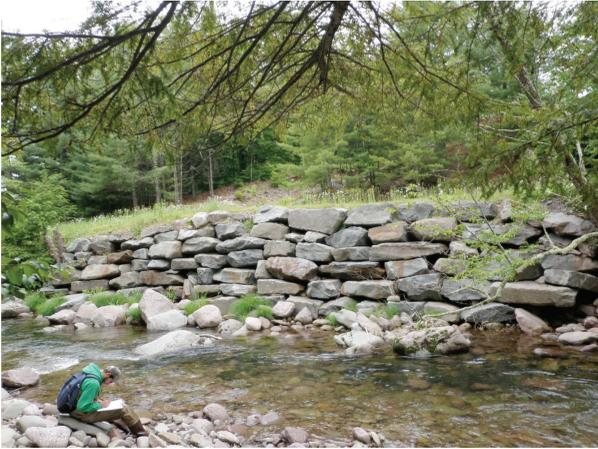
*Stacked rock wall on right bank protecting Denning Road (B152)*
