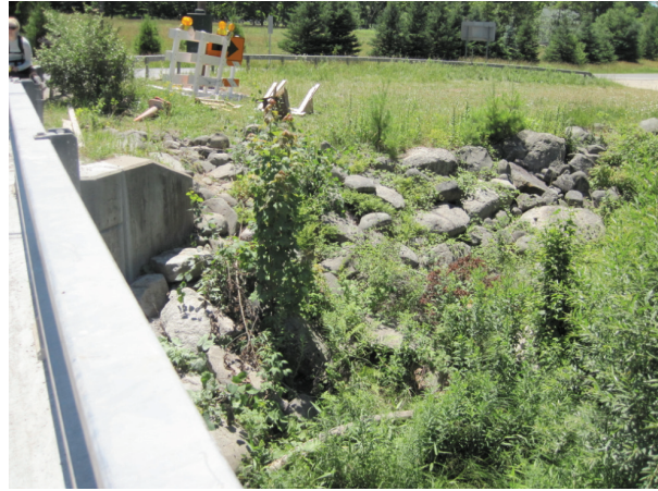
Left bank revetment at bridge abutment (A515)
