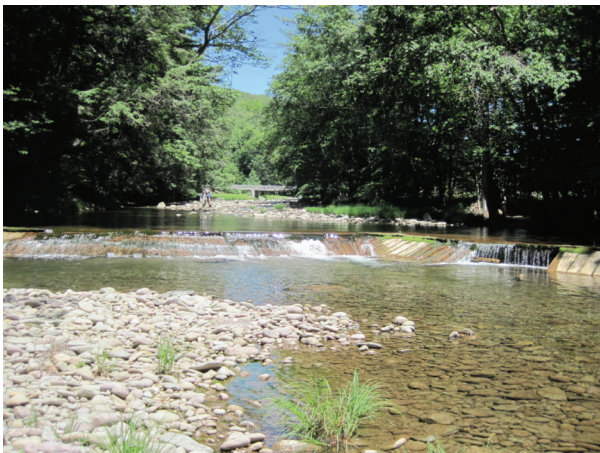
Timber dam spanning channel width (A522)
