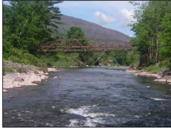
Bridge at Carr Road (Station 83957)
