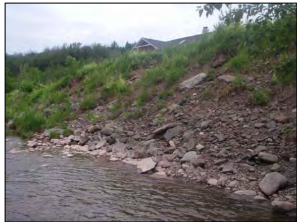
Bank erosion and planting site at Station 88000
