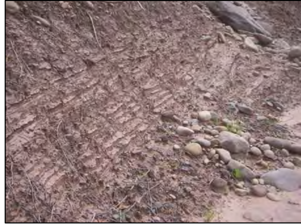
Clay exposure at Station 88900
