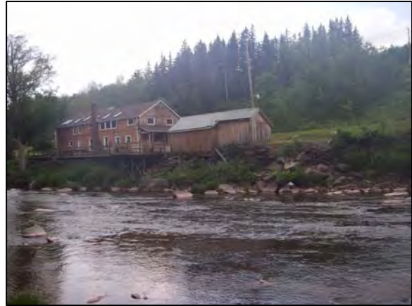
Stacked rock wall at Station 86250
