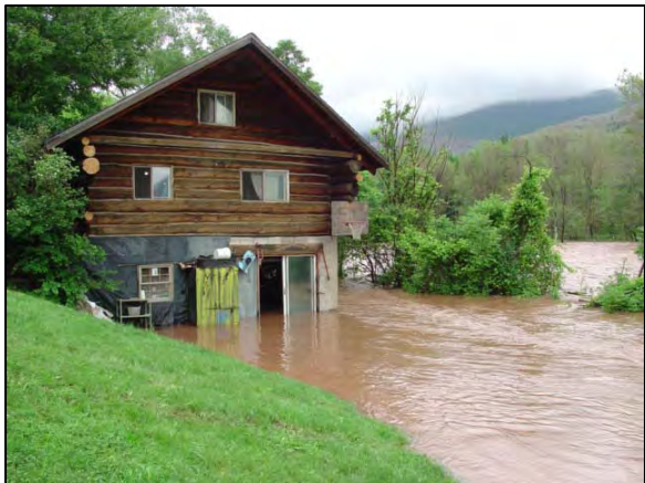
Flooding of residence at Station 84700
