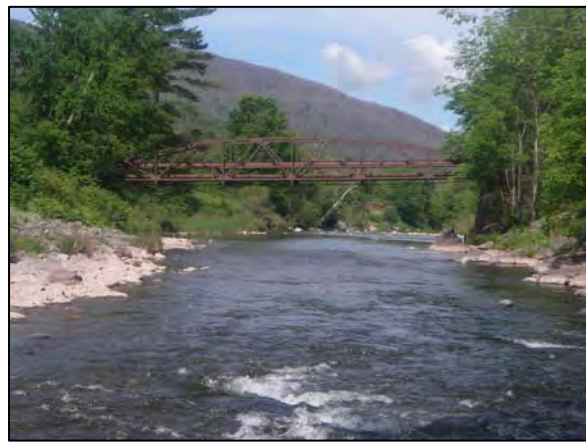
Bridge at Carr Road (Station 83957)
