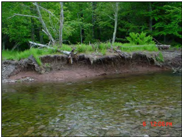
Clay exposure and bank erosion at Station 138500
