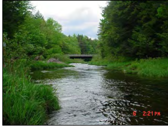
Bridge at Elka Park Road at Station 134100
