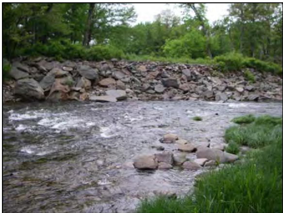
Rip-rap at Station 130850
