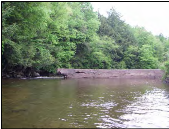
Dam remnants at Station 133700
