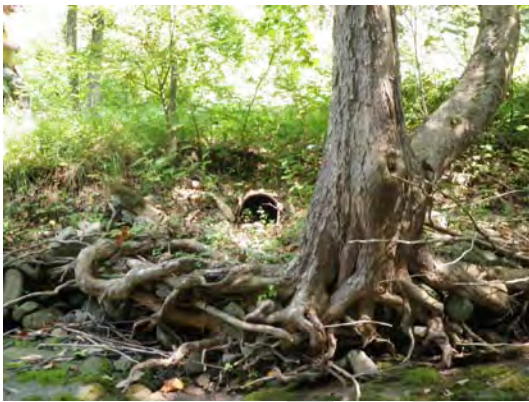
Figure 10 A smooth steel piped outfall through the right floodplain
