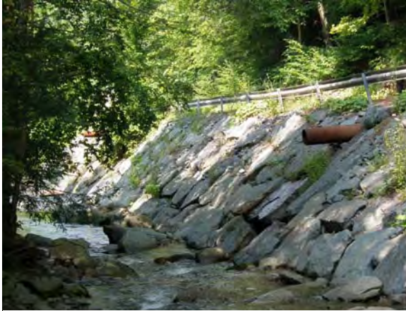
Figure 12 Tiled stone revetment, right bank, with two steel culvert outfalls visible
