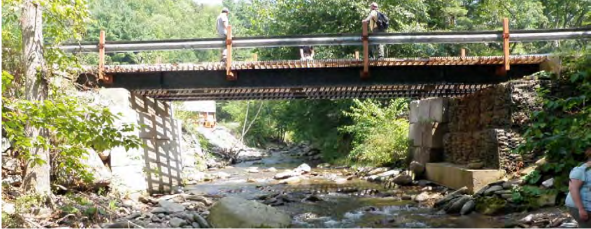
Figure 19 Sheely Road Bridge, Stn 1000, looking downstream
