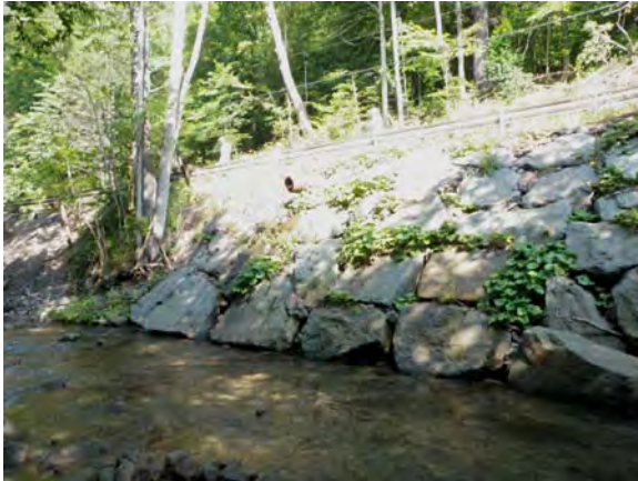
Figure 5 Tiled rock revetment at Stn 3300, Greenville Road embankment
