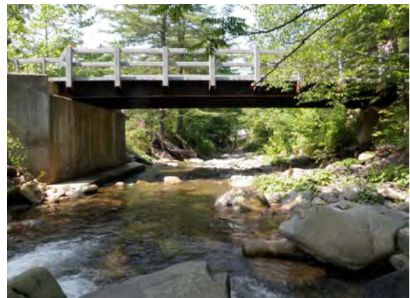
Figure 16 Bridge crossing at Stn 1600
