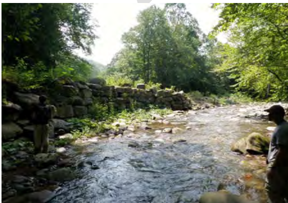
Figure 21 Revetment protecting Huttar Lane, Stns 500 to 800, looking DS, left, and US, right
