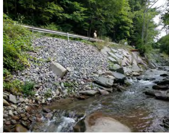
Figure 13 Dumped stone revetment, piped outfall in distance
