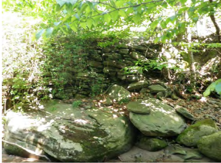
Figure 9 A stacked rock revetment on the right bank
