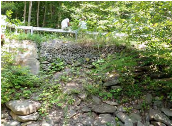
Figure 14 Gabion basket, right bank, near bridge abutment
