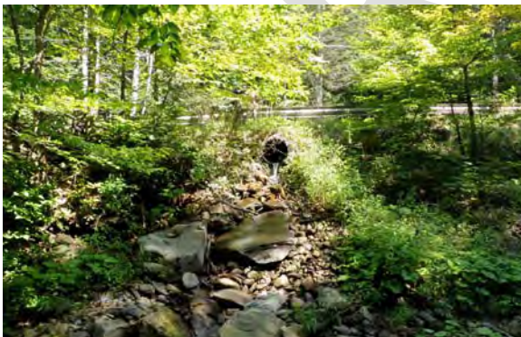
Figure 8 A plastic piped outfall, right bank
