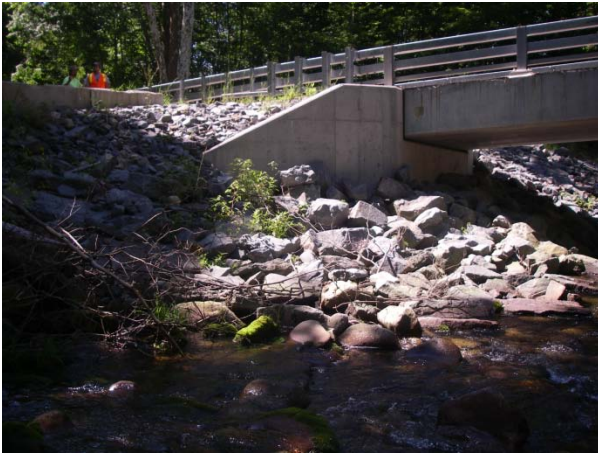
Figure 3 Abutment at Balace Road bridge evident here.
