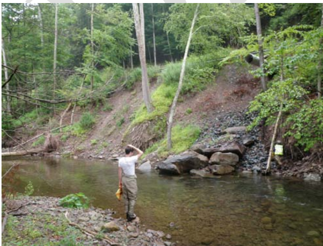
Figure 12 Erosion of embankment along Sundown Rd.
