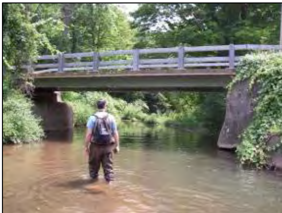
Champlin Road Bridge at Station 21930
