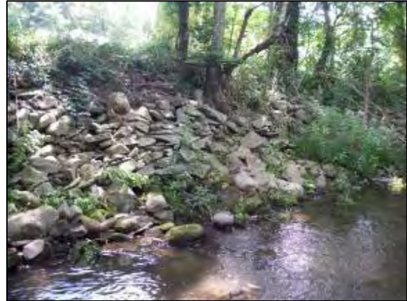
Revetment at Stations 22333
