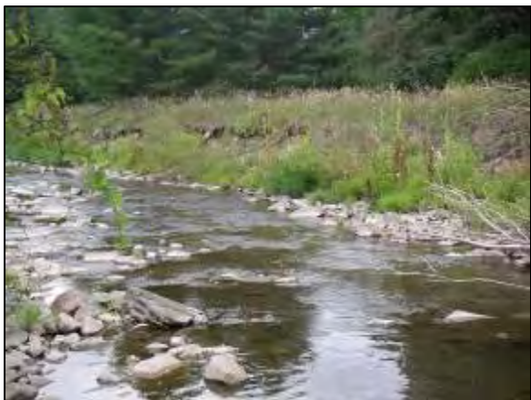
Erosion at Stations 20335 - 20124
