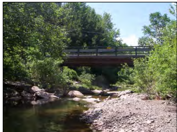
Vista Ridge Road Bridge at Station 67777
