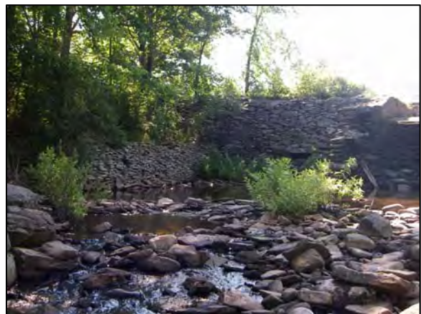
Rock wall at Station 73728
