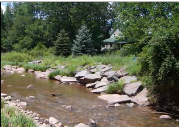
Rip-rap along right bank at Station 68717
