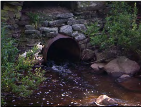
Culvert at toe of dam, Station 73728
