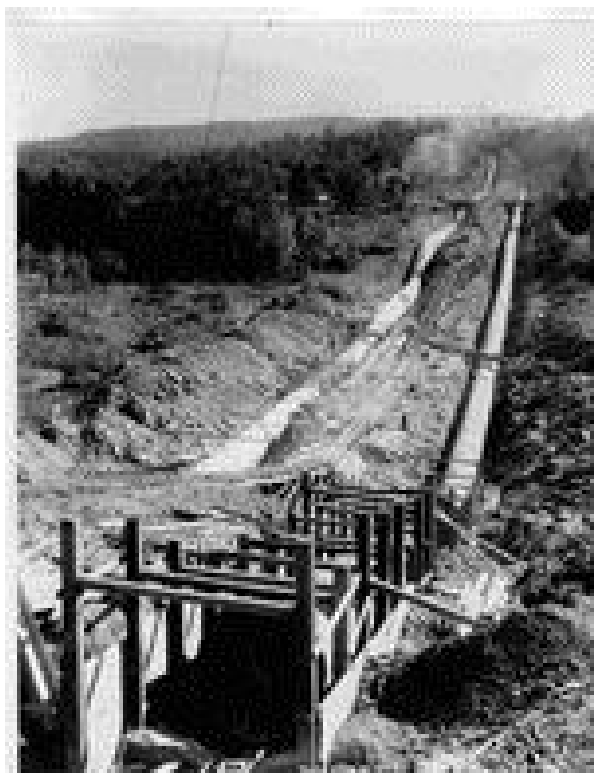
Photo 3. Catskill Aqueduct. October 3, 1923 (NYC DEP, 2003).
