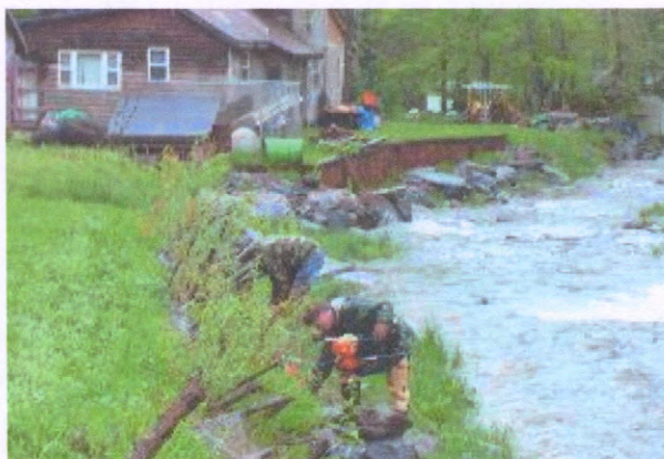
Photo 14. Trout Unlimited volunteers assisting bioengineering efforts along the left bank of MU3, looking downstream, riparian planting day, May 18, 2002.
