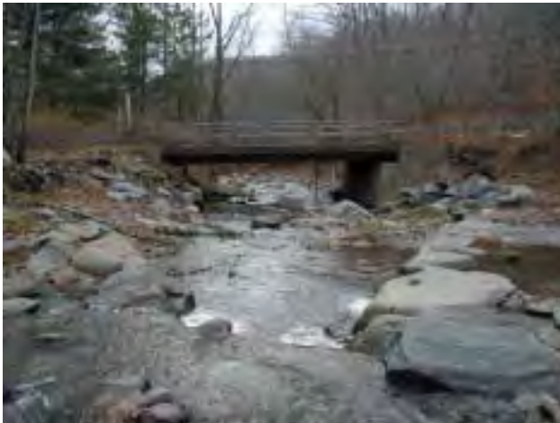
Photo 8. Looking downstream at County Bridge 3201240, at the bottom of MU3.
