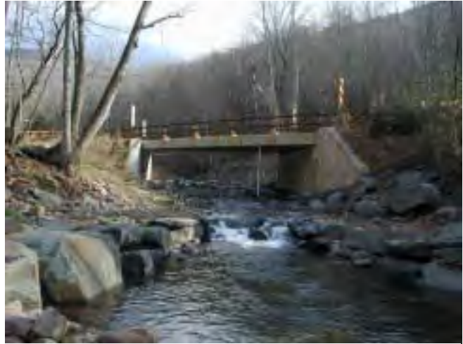
Photo 7. Looking upstream at County Bridge 3201230, at the top of MU3.
