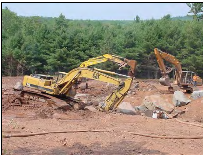
Figure VII-19: Construction of rock structures at the Big Hollow site.
