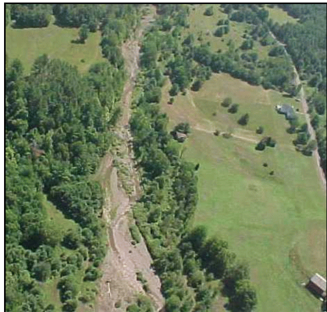
Figure VII-17: Preconstruction aerial view of Big Hollow site, note the braided channel at bottom, and lack of sinuosity at top.
