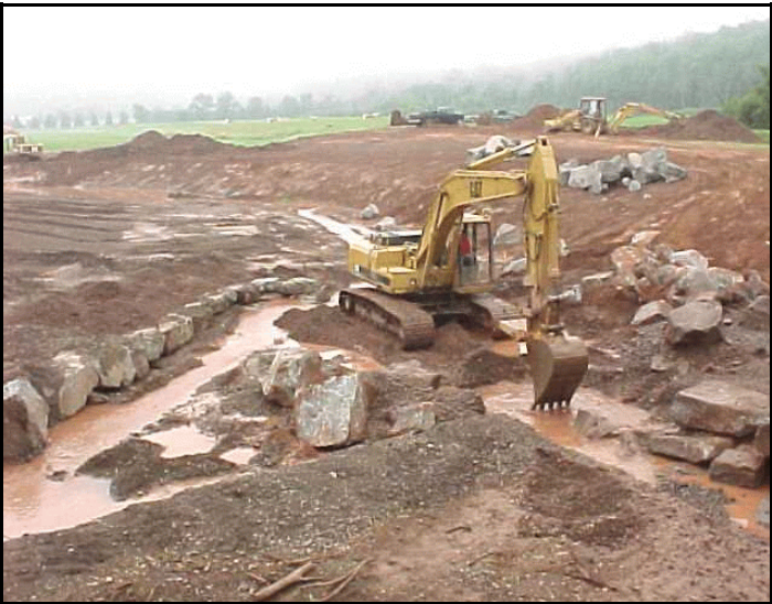
Figure VII-12: Construction of w-weir.
