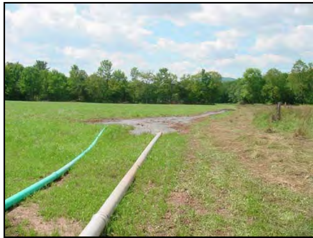
Figure VII-4: Sediment-laden water is pumped to grassy fields for settlement of solids.
