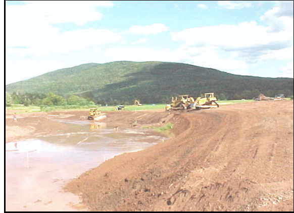
Figure VII-5: Extensive grading was required to create the new channel form.
