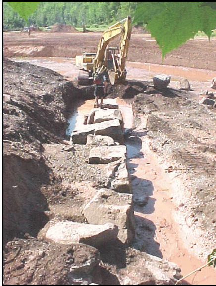
Figure VII-6: Construction of rock vanes proceeds after the channel is graded .
