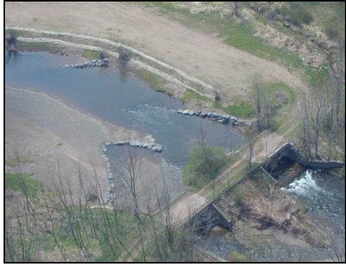
Figure VII-13: Aerial view of completed w-weir
