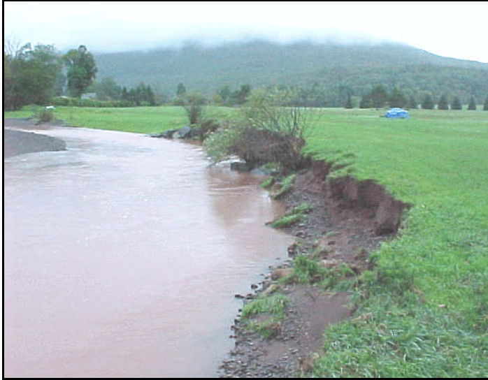
Figure VII-22: Erosion on upper streambanks after tropical storm Floyd. The lower toe of bank remained unchanged.
