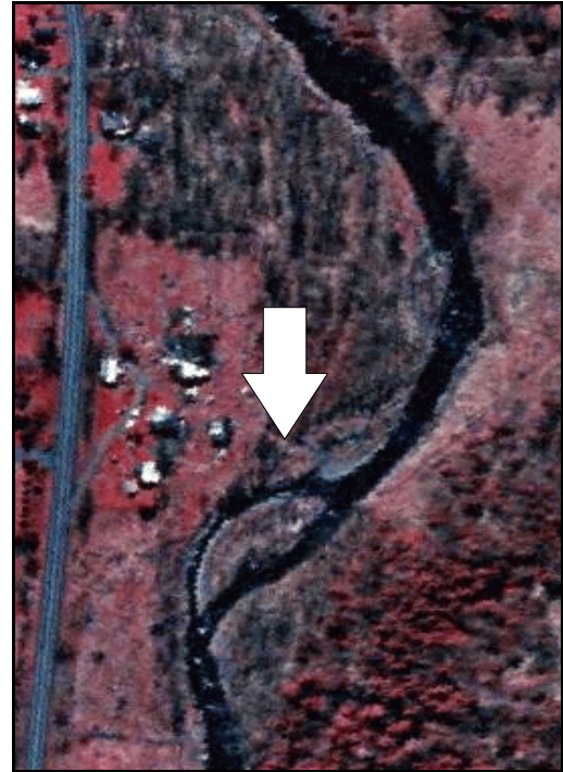
Figure VI-92: 1995 aerial of lower end of reach 5c. Note split channel in location of former bridge.
