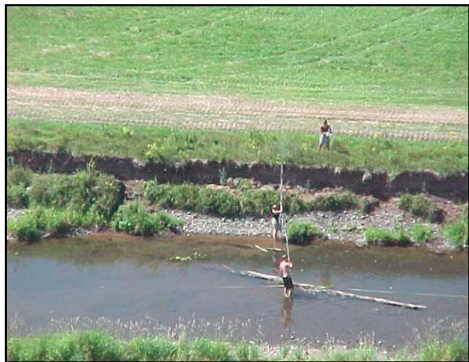
Figure VI-54: Eroding streambank on Maier Farm property prior to restoration.
