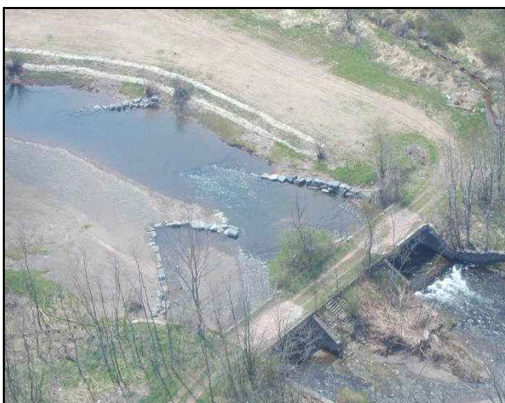
Figure VI-58: View of private bridge on Maier Farm post restoration work. Note the two openings with the large, solid center section.
